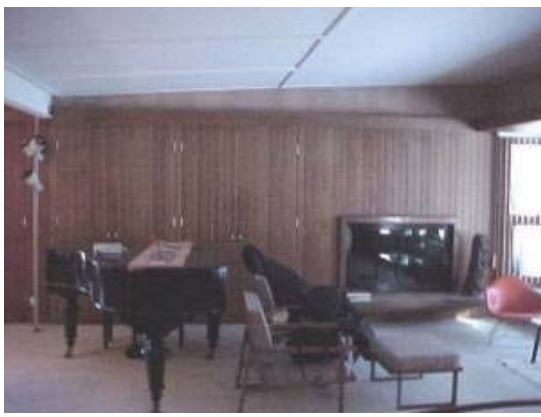
Close House Living Room before Renovation
