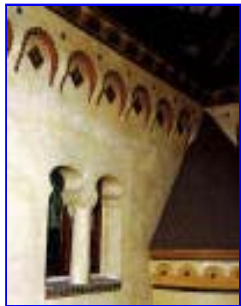
Upper Wall: Hall of Records
